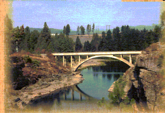
Post Falls Bridge
